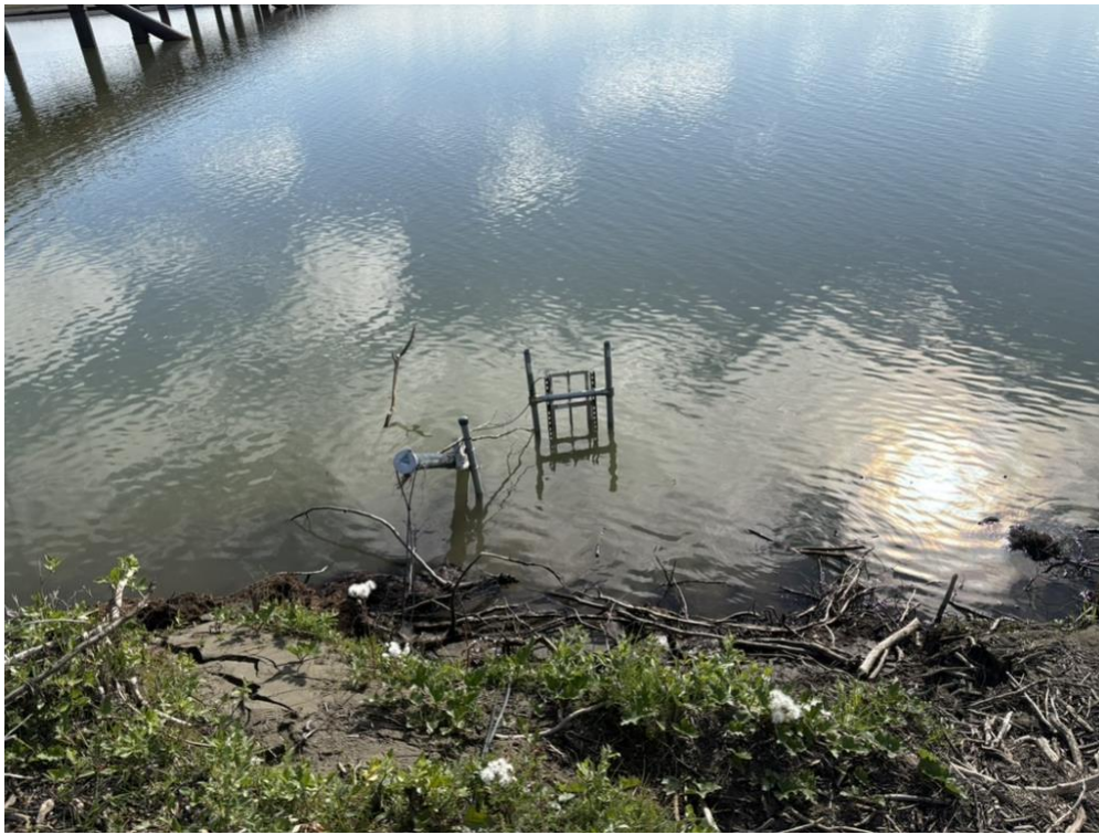
Figure C.10. Mid-installation view showing sensor frame placement and mounting alignment along the channel bank. (NVN DNR, 2025)
