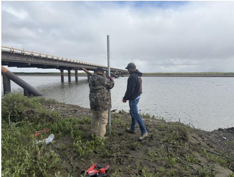
Figure C.8. Installation of the main support pole using hand post drivers to ensure secure anchoring into the riverbank substrate. (NVN DNR, 2025)
