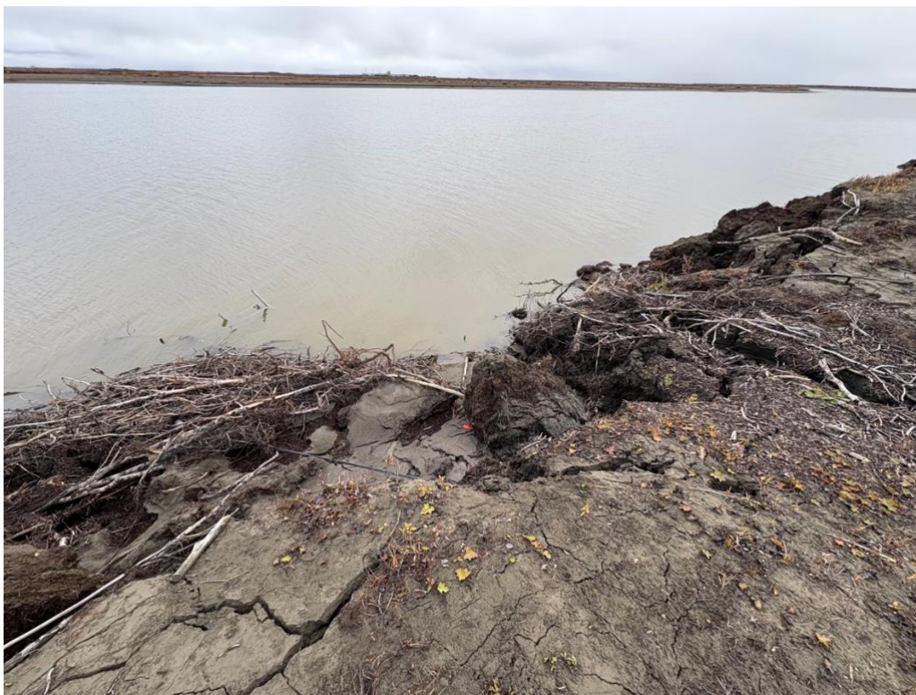
Figure C.22. Collapsed tundra edge and exposed permafrost near the Niquiq Bridge installation. Tilted sensor ladder visible in water. (NVN DNR, 2025)
